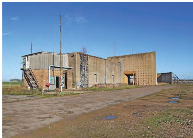
K 2 stand used to test horizontal rocket motors
